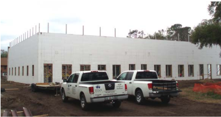
Above – 20ft high Amvic walls with 43 openings
